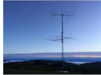
Top beam with Yaesu rotor 10-4/15-3/20-3 - 1 coax 40-2 - 1 coax
