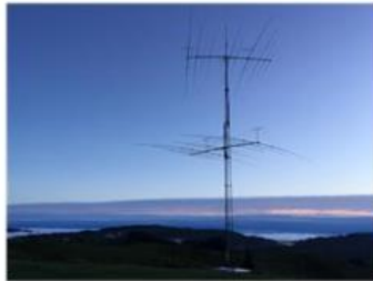
Top beam with Yaesu rotor 10-4/15-3/20-3 - 1 coax 40-2 - 1 coax
