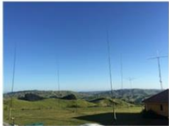
80 m 4 square with DX engineering coupler Position OMNI - omnidirectional Position 1 - 330 degrees = AS, EU-SP Position 2 - 60 degrees = NA/Caribbean Position 3 - 150 degrees = SA/EU-LP Position 4 - 240 degrees = VK/ZL not much more
